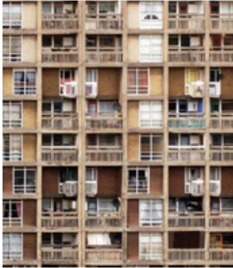
Fig 2.89 The original Park Hill façade, with brickwork infill and single-glazed units
