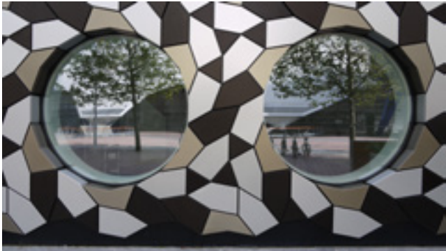
Fig 3.36 Tessellated anodised aluminium cladding panels, silver, bronze and champagne anodising, of Ravensbourne College
