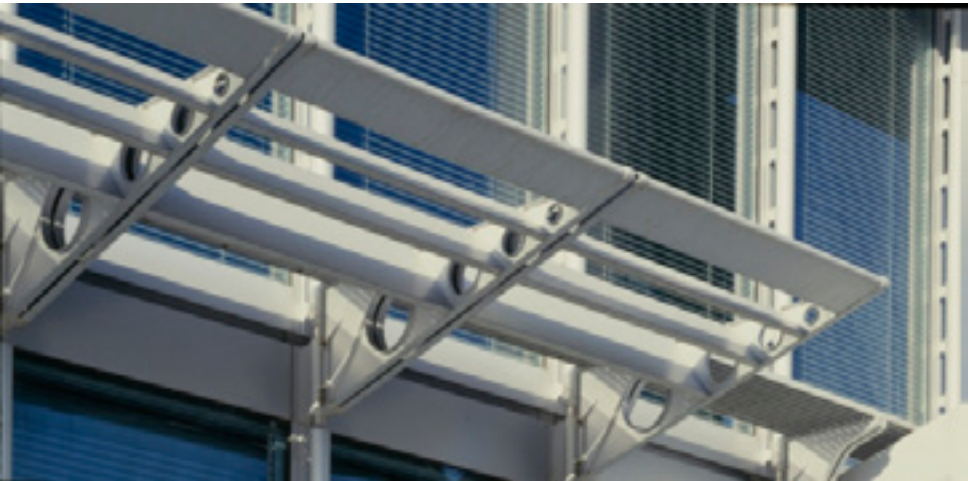
Fig 6.15 Brise soleil of the curtain walling of the Hongkong and Shanghai Bank Headquarters
