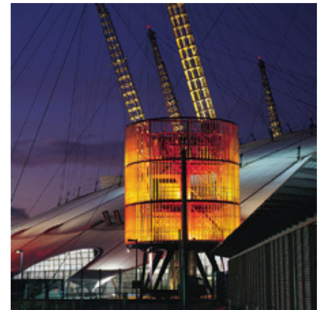
Fig 3.34 Extruded aluminium louvres clad the service pods – a total of 12 are located around the base of the Dome's canopy
