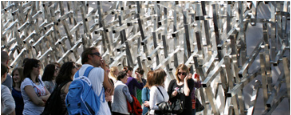
Fig. 2.2 Vague Formation, a mobile music pavilion designed by soma has an extruded aluminium structure
