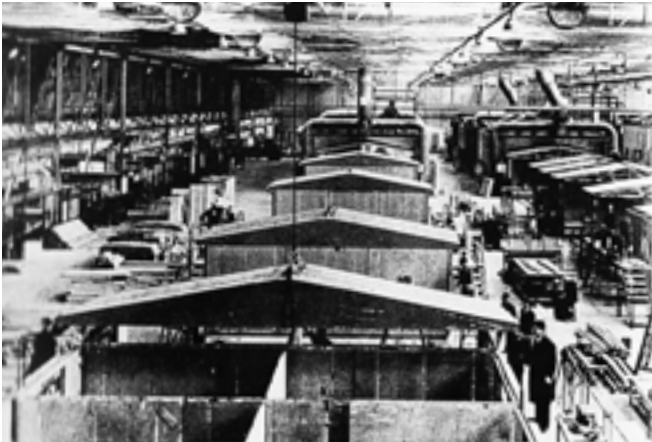
Fig 4.4 Factory production of AIROH aluminium homes in prefabricated segments
