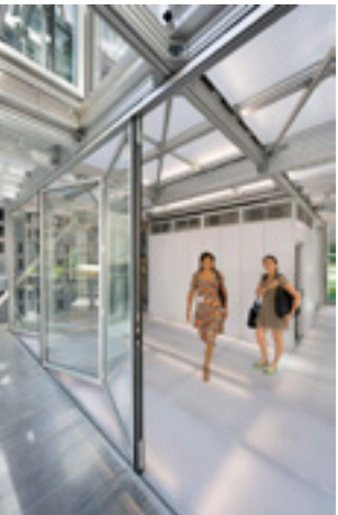
Fig 4.72 Folding glass doors to the terraces of the house provide access and natural ventilation
