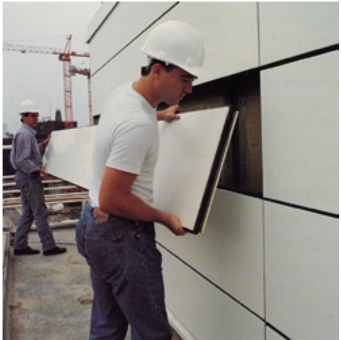
Fig. 2.47 Aspect 2 cladding system installation
