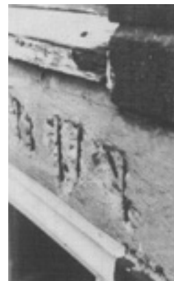
Fig 2.71 Parsons House before renovation – note the spalling concrete and rotten timber windows
