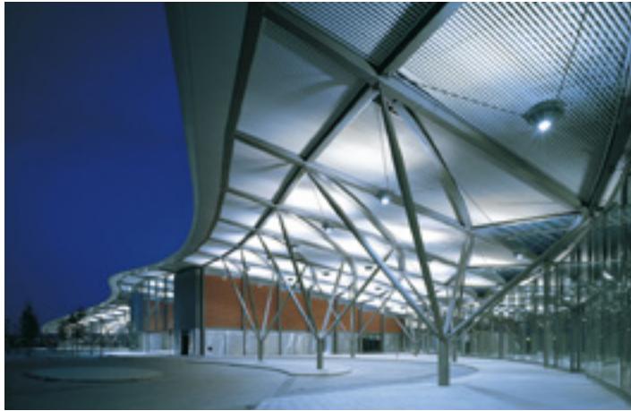
Fig 3.28 Architect Foster + Partners' North Greenwich Transport Interchange has an aluminium standing-seam roof
