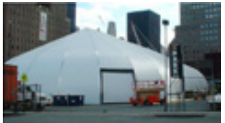
Fig 4.17– Fig 4.20 Sprung-tensioned membrane fabric structures, which have a lightweight aluminium frame and perform well in all climates, from the ‘Ground Zero’ construction site to the Arctic Watch Wilderness Lodge
