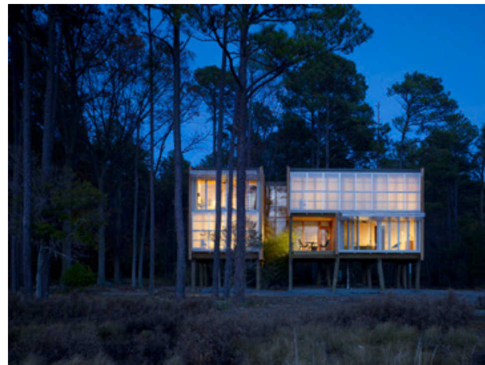
Fig. 2.41 The Loblolly House, designed by KieranTimberlake, is an example of reversible construction, which uses Bosch Rexroth aluminium extrusions
