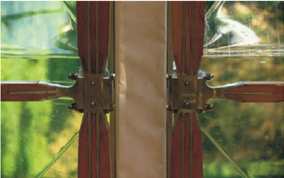
Fig 4.61 Flexible polymer movement joint between two timber, aluminium and polycarbonate arches
