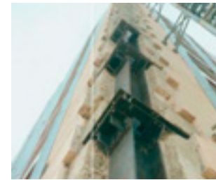
Fig 2.64 Corroded steel frame of the Empire State Building during renovation
