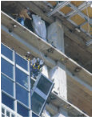
Fig 2.54 Replacement of the panelised curtain-walling system of the UN Secretariat Building in 2007
