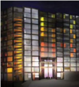
Fig. 2.50 Park Hill at night, incorporating anodised aluminium panels as part of redevelopment by architect Hawkins Brown and Studio Egret West
