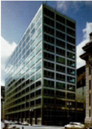
Fig 6.2 The Equitable Building, Portland, Oregon, designed by Pietro Belluschi, incorporates cast aluminium cladding panels
