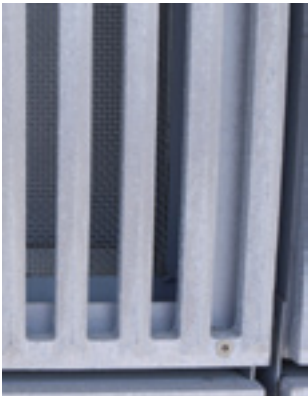
6.21–6.22 Cast aluminium solar shading of Heelis
