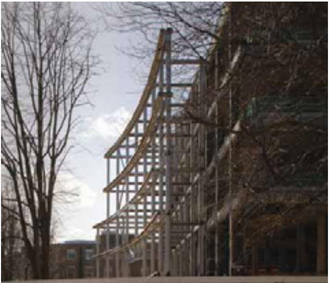
Fig 2.85 The steel frame, which extends from the existing concrete frame
