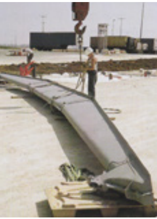
Fig 4.47– Fig 4.51 The beams being restored, ready for reassembly in Villepinte
