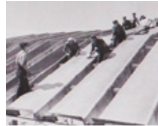
Fig 4.31 Aluminium panels being attached to the pavilion structure in Paris
