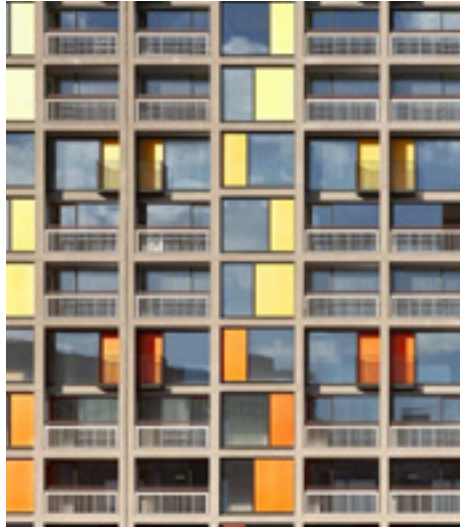
Fig 2.90 The Park Hill façade after refurbishment, with double glazing and coloured anodised aluminium infill panels
