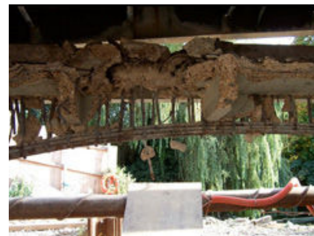
Fig. 2.12 The 1911 Ballingdon Bridge being demolished in 2002, with both the concrete and mild steel reinforcement about to be recycled
