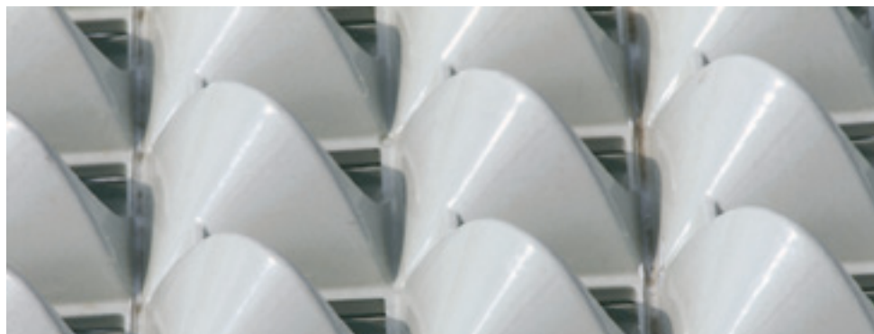
Fig 6.17 Cast aluminium shells of the solar shading at the Nasher Sculpture Center, designed by Renzo Piano Building Workshop
