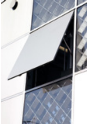
Fig 5.19 A flush detailed ventilator articulates the 1200 mm module of this prototype Aluminium House in Kyushu, Japan, designed by architect Riken Yamamoto & Fieldshop
