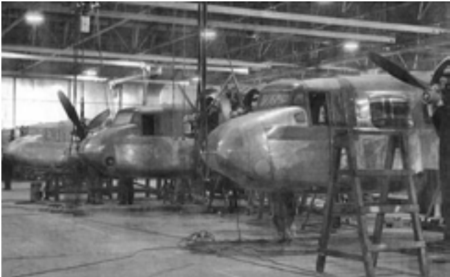
Fig 4.3 Aluminium plane production at the Blackburn Aircraft factory during the Second World War
