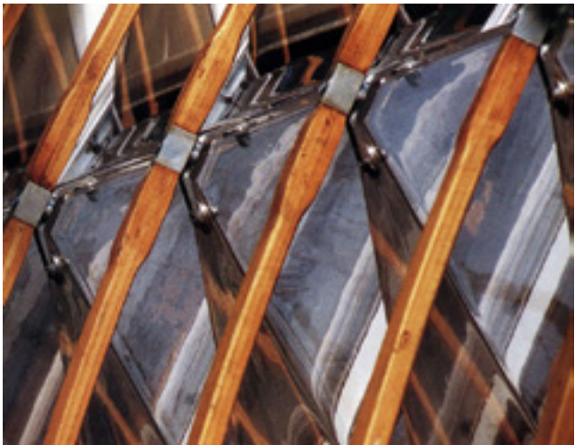
Fig 6.11 Cast aluminium nodes linking shapely timber sections with the structural polycarbonate skin
